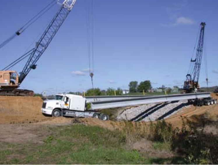
Cranes lower the third girder into position next to the first two girders placed, sequencing the placement from west to east.
